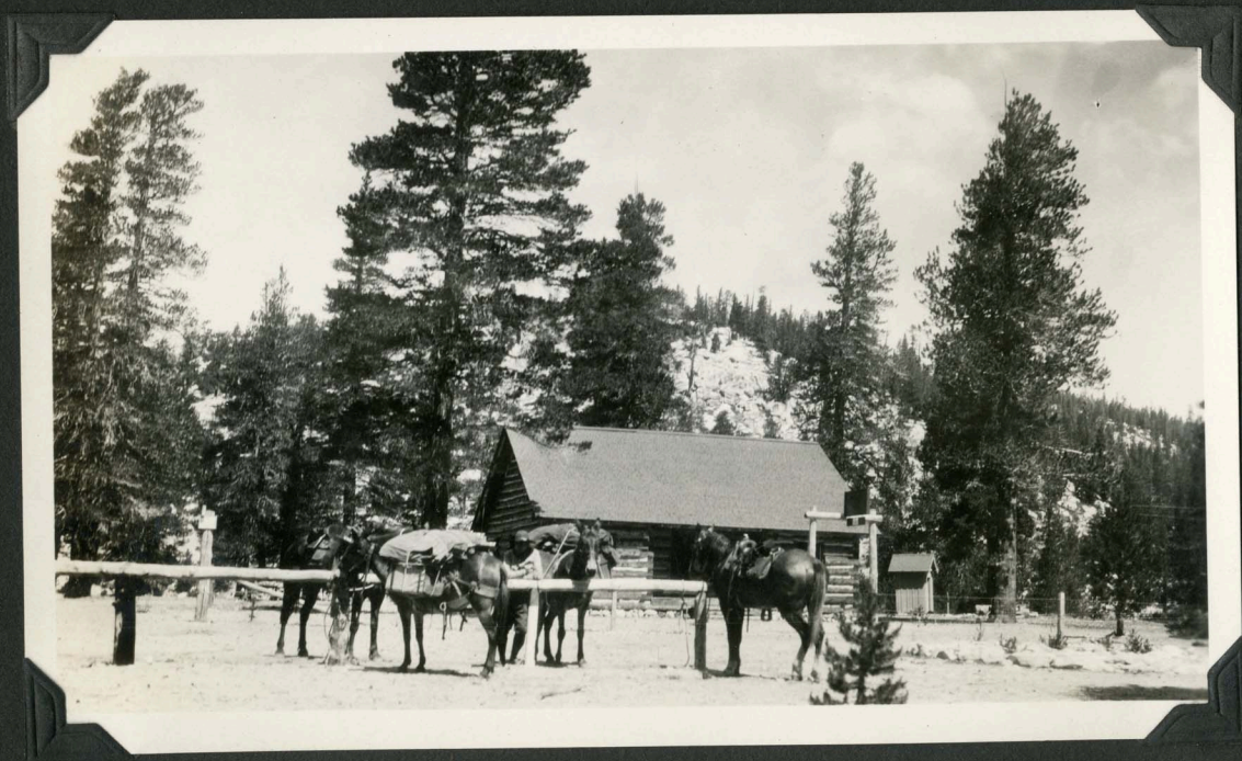
Tunnel Ranger Station
