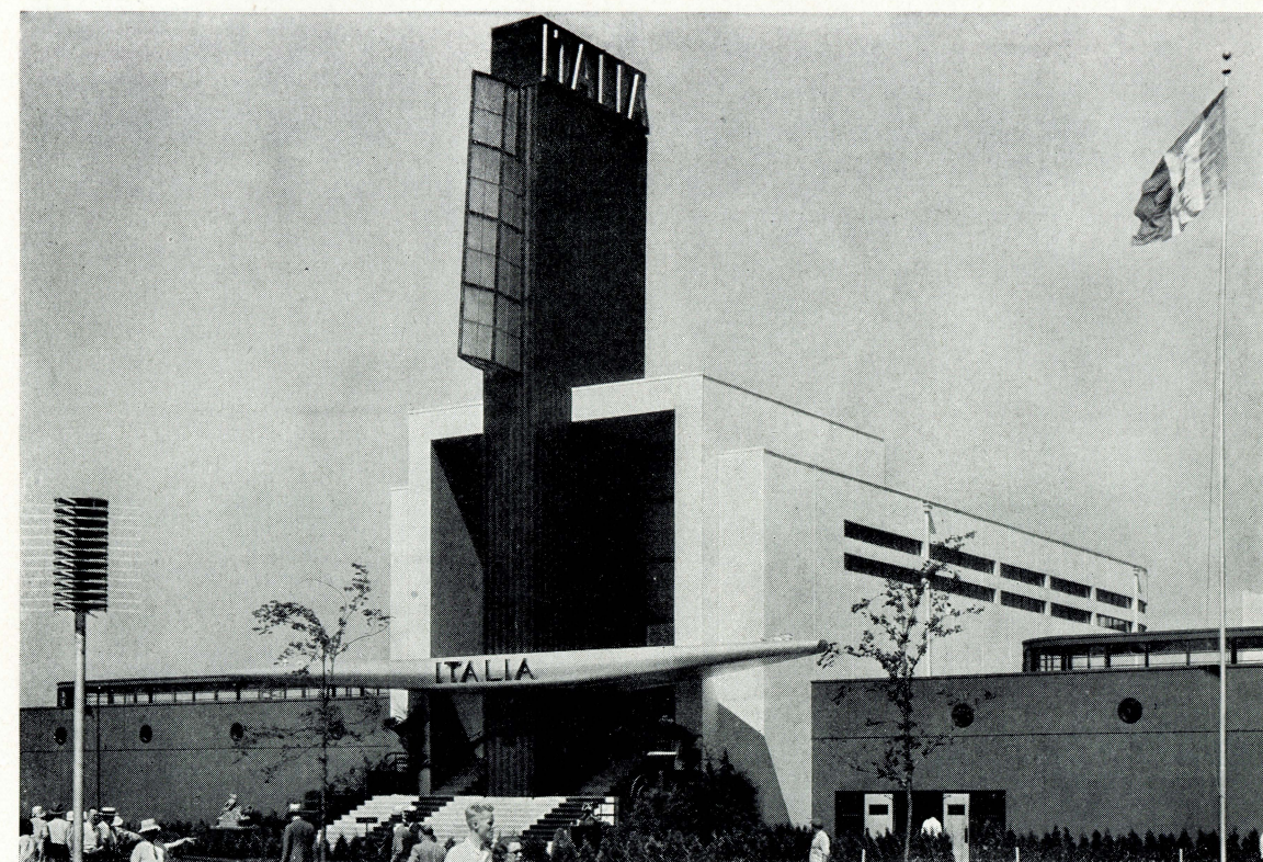
The Italian Building
