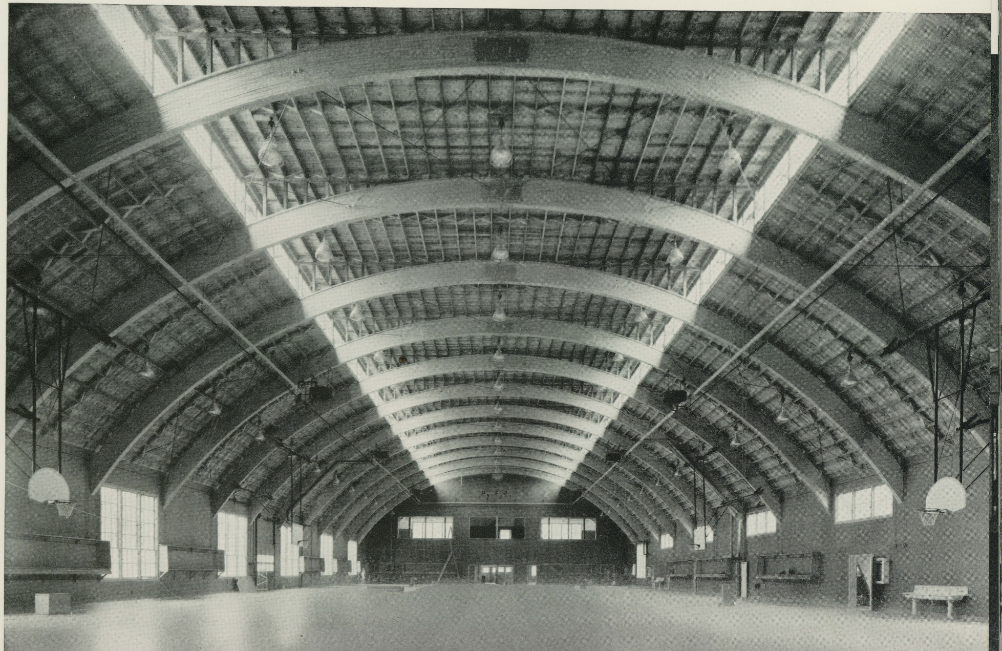
→ Drill hall interior, showing laminated arch construction.
