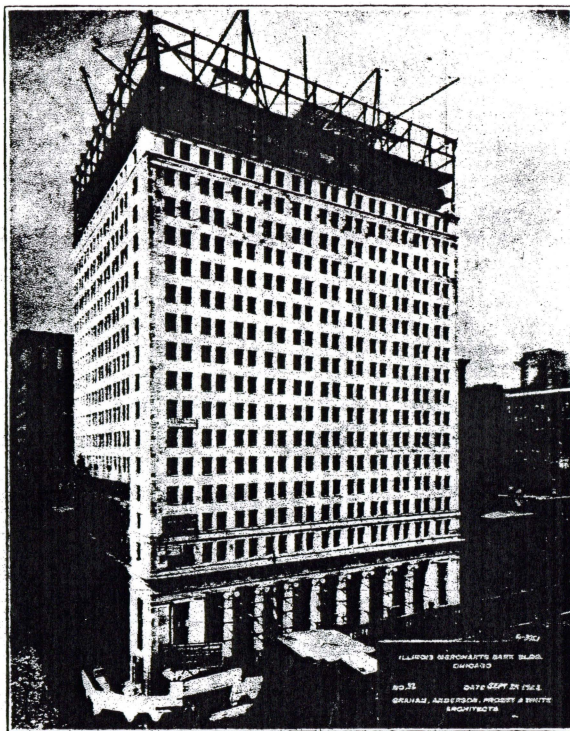
Finishing Exterior Work on Huge Bank Structure. (Courtesy American Contractor.)
